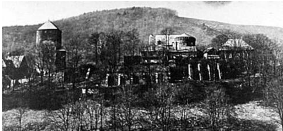
Figure 2. Burg Altena as it appeared before renovation around the turn of the 19th century. This image of the castle is from the Universität Gesamthochschule Siegen , where it was described as having badly deteriorated at the time this photograph was taken.
